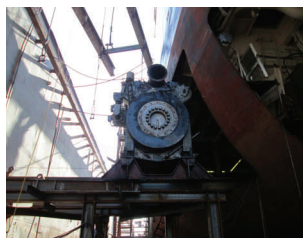
Cooper 16 Cyl Propulsion Engine on rails outside the hull. Weight Approx. 50 Ton
